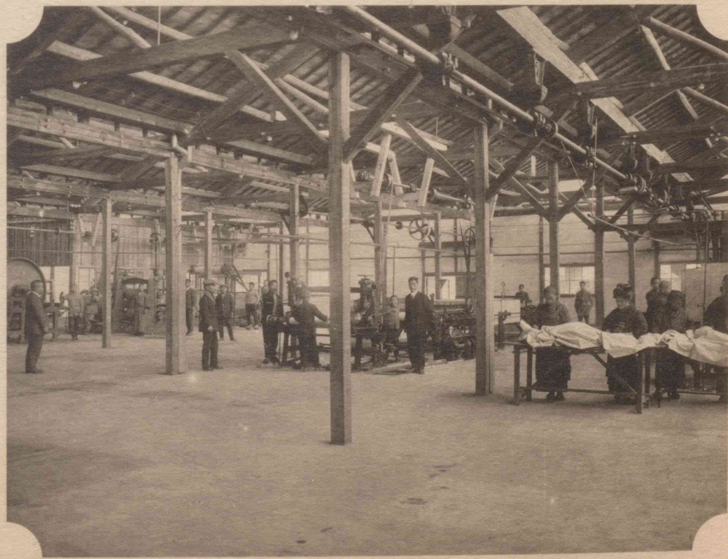
部一ノ場工上仕 A Portion of the Finishing Works.
